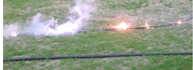
Fig. 21: Overhead line on meadow
