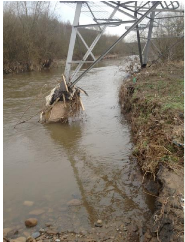
Fig. 3: Foot of tower 132kV following movement of river
