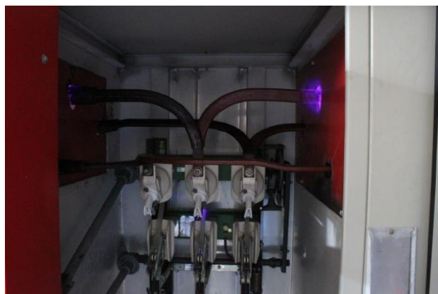
Figure 4 from paper 0665: AIS equipped with switches and a busbar in ambient air – Corona effect around the busbar going through the insulating plate and on the insulating rod of the switch
