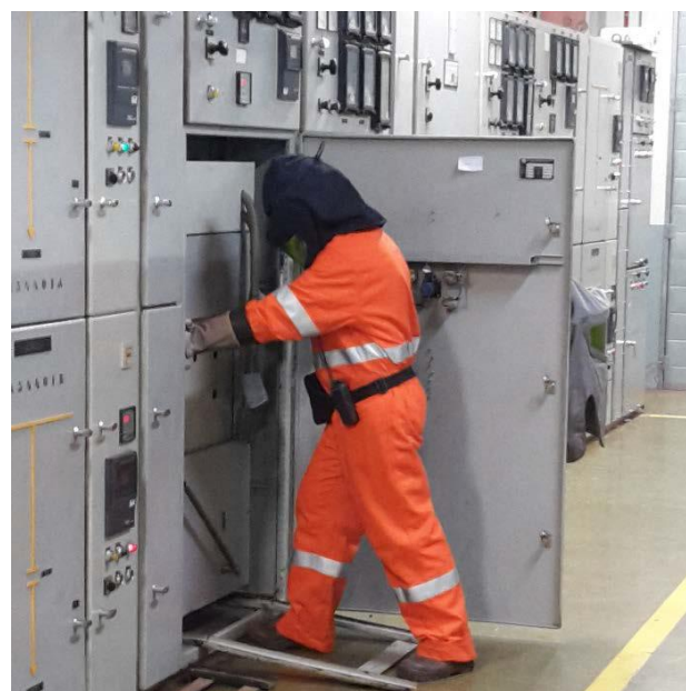
Figure 1 from paper 0796: Open-door circuit breaker racking-in operation
